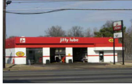
Inappropriate Roof Screening
